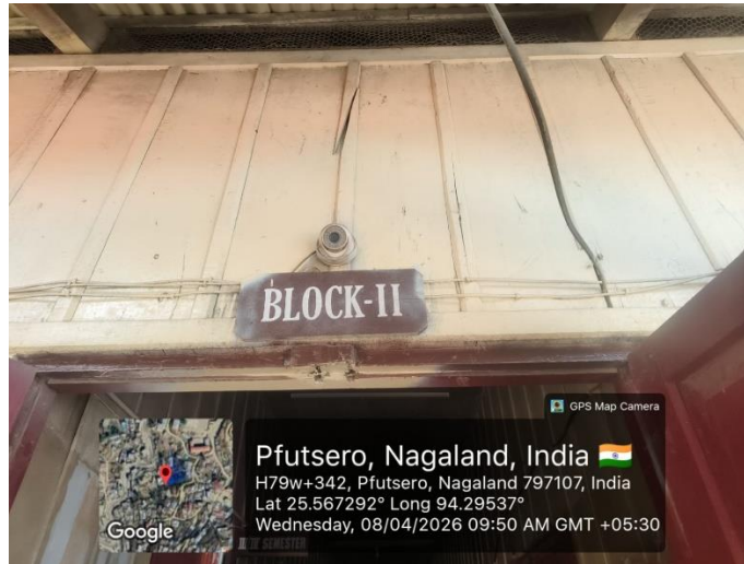
CCTV cameras at strategic locations
